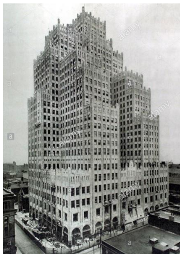
Figura 7 – Edifício Southwestern Bell Telephone Company
