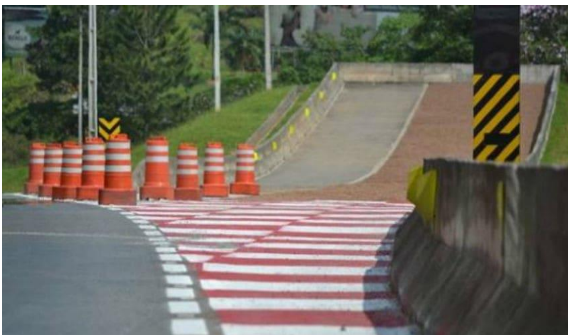
Figura 01 – Rampa de escape [CBN Curitiba]
